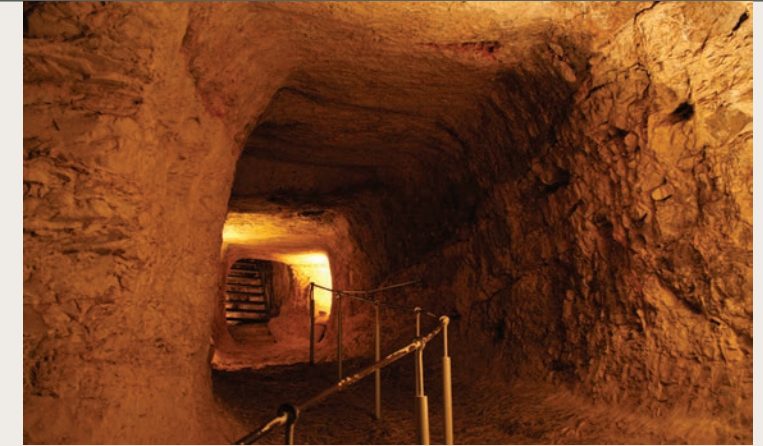
Part of the underground water tunnel that leads from inside the city of Jerusalem to an outside water source. At the end of the tunnel is a 43 1/2-foot shaft that drops down to the Gihon Spring. The tunnel system provided the people of Jerusalem access to water, even when the city was under attack from outsiders.
